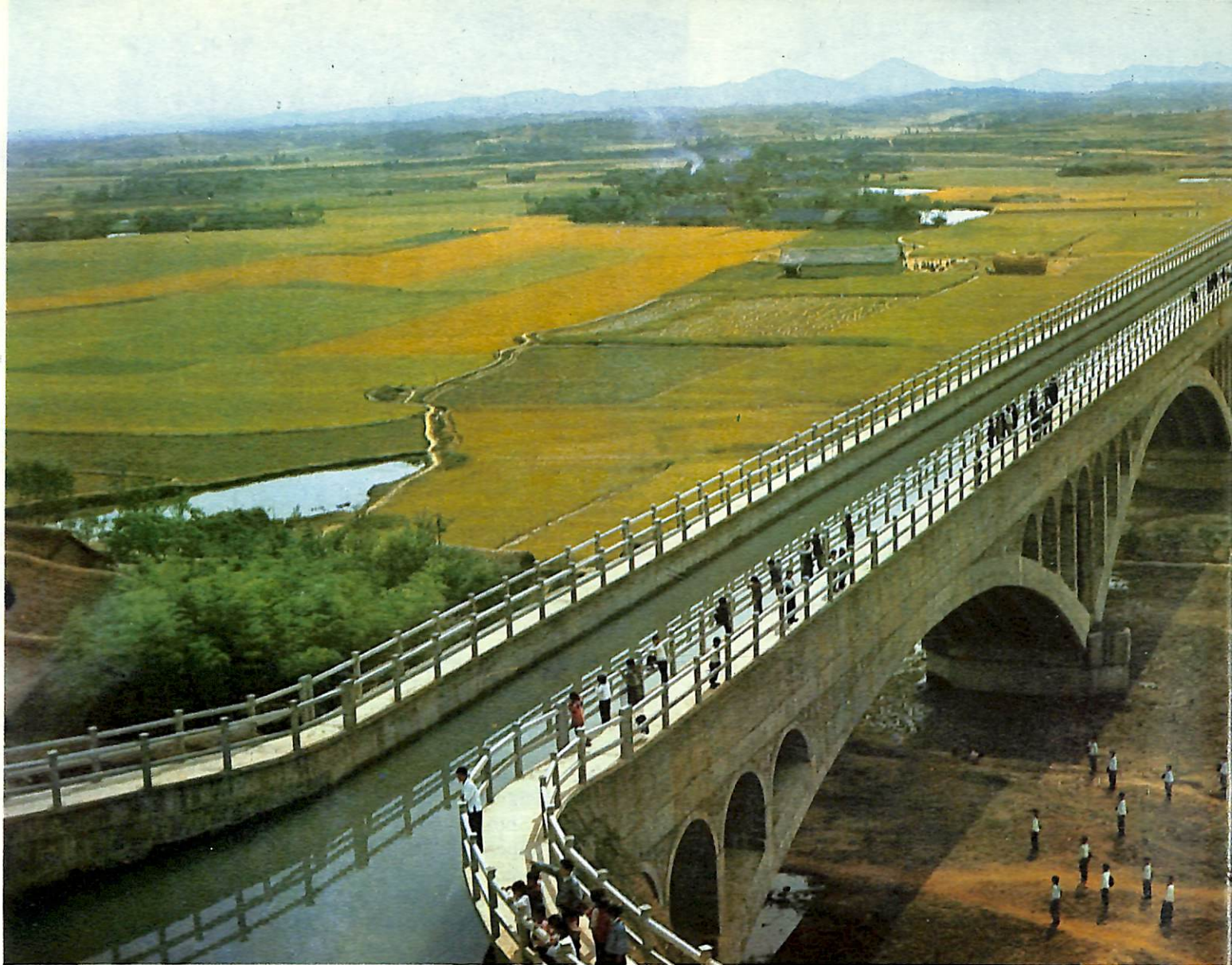
The Chiangchunshan Aqueduct.
